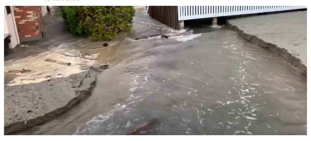
This breach was Fixed with a permitted repair to the existing Soft shore, the sheet pile was left elevated with a cap on it. The primary shoreline protection is the anchored log soft shore.
